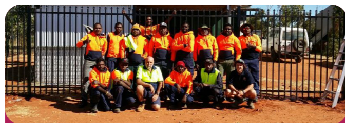
Yuendumu Recycling Shed, Central Desert Regional Council, Northern Territory: A seven-bay recycling shed has been built using government grant funding and is designed to introduce recycling to the community. It enables the community to drop-off of bottles, tyres, gas bottles, motor oils, paints and chemicals, batteries and white goods.
